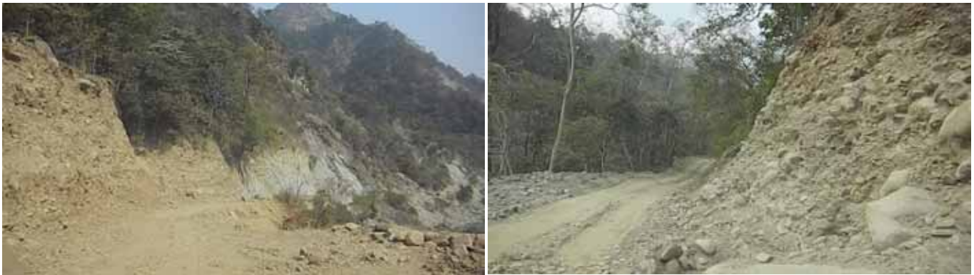
Hill side cutting in progress
